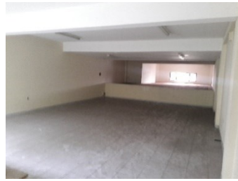
Figure 22: Lounge before the refurbishment, 2016
