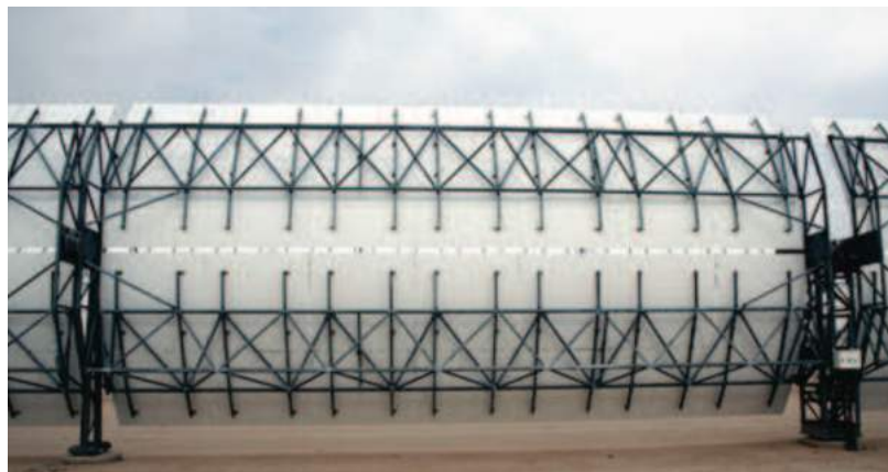
Figura 2.10 – Coletor solar LS-3. Fonte: Parabolic Trough CSP Technology: state of the art and market overview
